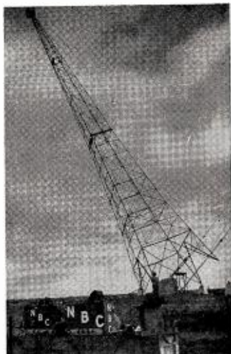
SPOT description of a station felling one of its own antenna towers was piped to listeners of KNBC San Francisco from Belmont, Calif. Station's remote unit (foreground) aired broadcast as the giant tower began to topple. Tower, one of two structures, was torn down to be replaced by a 550-ft vertical radiator antenna now under construction.
